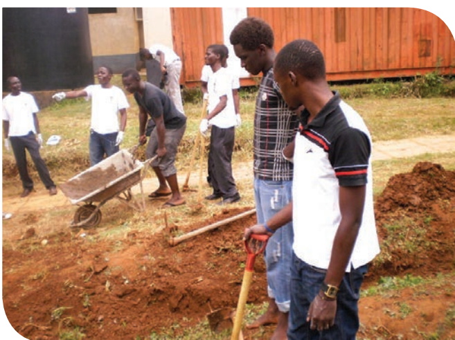
Desilting a drainage channel at the Kampala School for the Physically Handicapped in Ntinda
